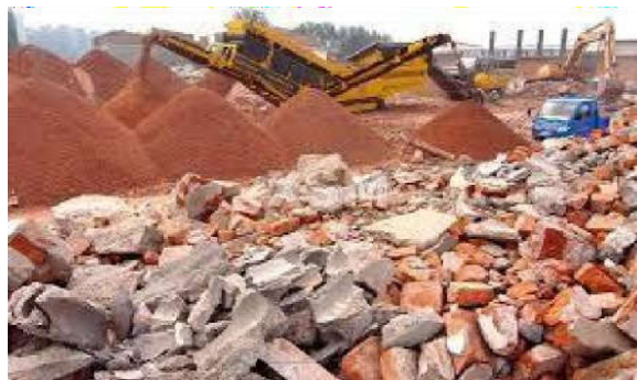
Fig. 3: Construction Demolition Waste
